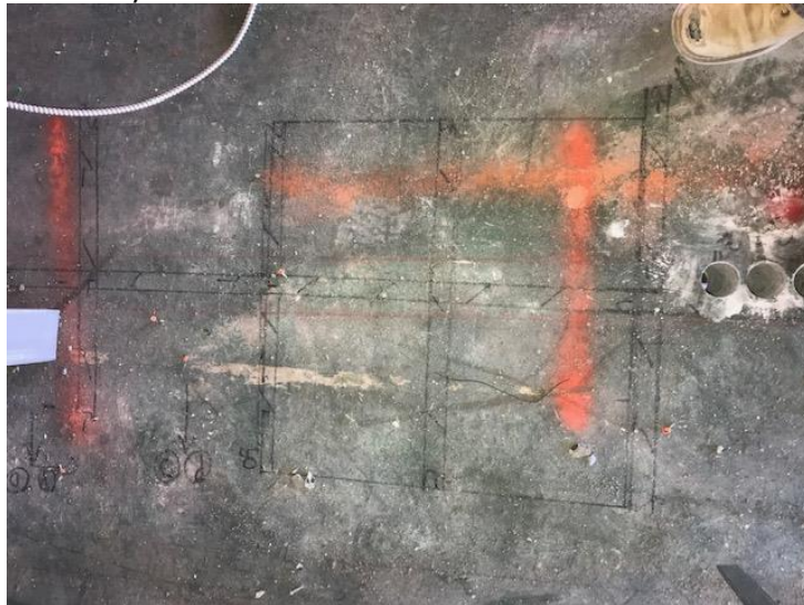
Scan #3/ Denoted at 09: This scan shows an 8" slab with top layer of rebar.
