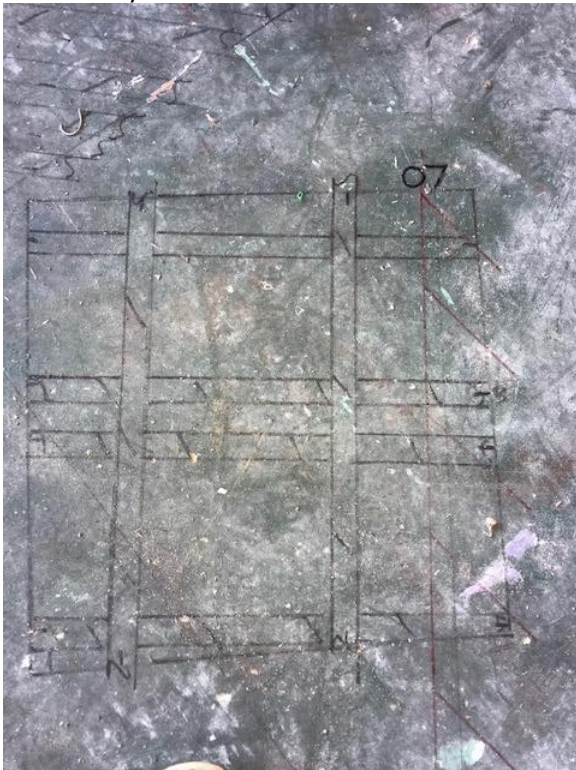
Scan #11/Denoted as 07: This scan shows an 8" slab with top and bottom layers of rebar. This scan abuts a post-tension beam and was marked in red, to avoid.
