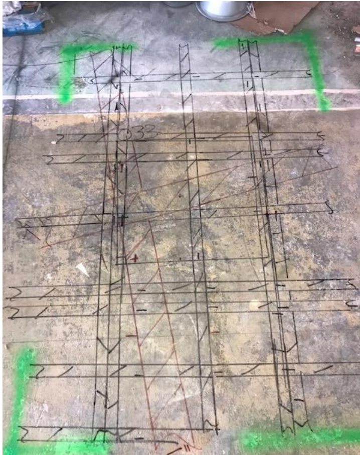
Scan #26/Denoted as 033: This scan shows an 8" slab with top and bottom layers of rebar, a two possible conduits or cables, at a depth of 7" running horizontally through the slab.
