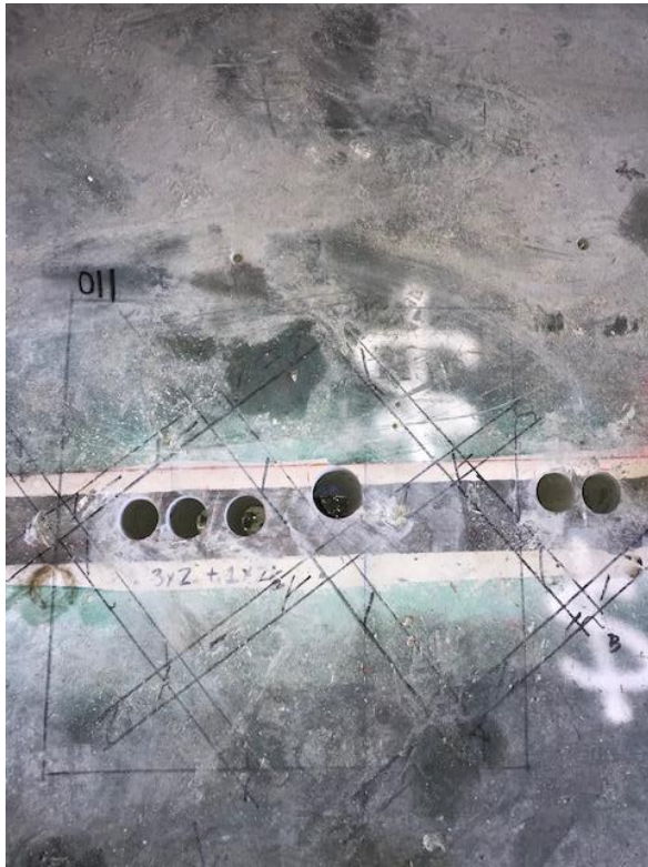
Scan #7/Denoted at 011: This scan shows an 8" slab with top and bottom layers of rebar.
