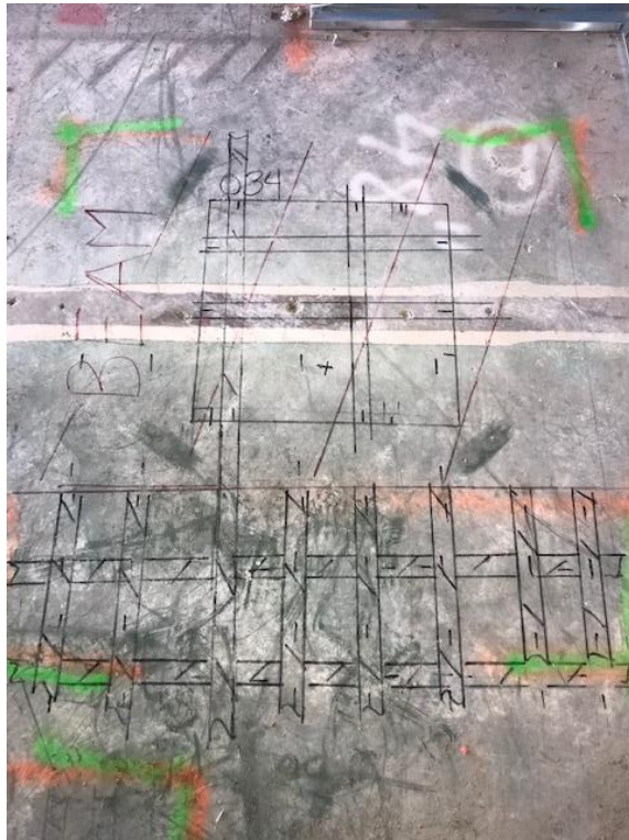
Scan #30/Denoted as 034: This scan shows an 8" slab with top and bottom layers of rebar, abutting a post-tension beam, marked in red to avoid.
