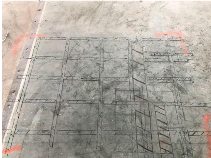
Scan #41/Denoted as 010: This scan shows an 8" slab with a top and bottom layer of rebar, with a possible conduit or cable at a depth of 3", and a second target anomalous target at a depth of 6", both of which were marked in red to avoid.
