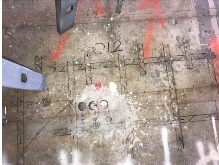
Scan #43/Denoted as 012: This scan shows an 8" slab with a top and bottom layer of rebar.
