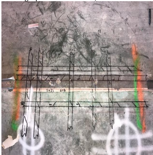
Scan #31/Denoted as 007: This scan shows an 8" slab with top and bottom layers of rebar.
